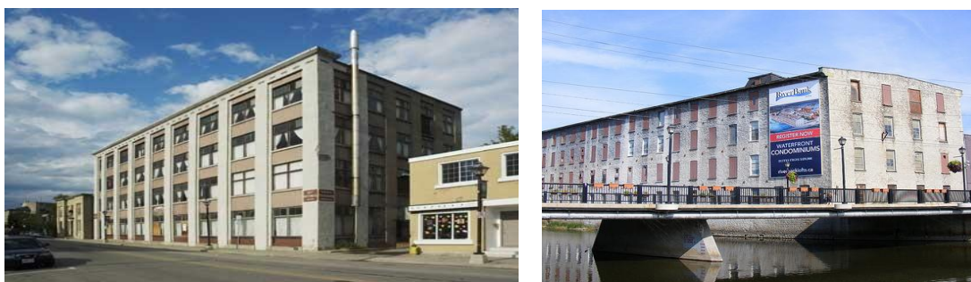
New Condominiums located in Cambridge: Tiger Brand building in downtown Galt and Riverbank Condominiums on Speed River in Hespeler.
